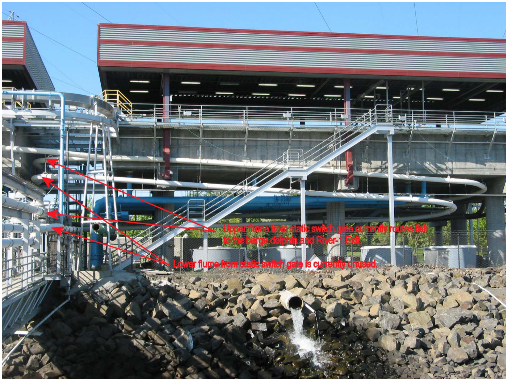
This shows the routes of the two available pipes downstream of the static switch gate as they loop around under the West Raceway banks at McNary.
