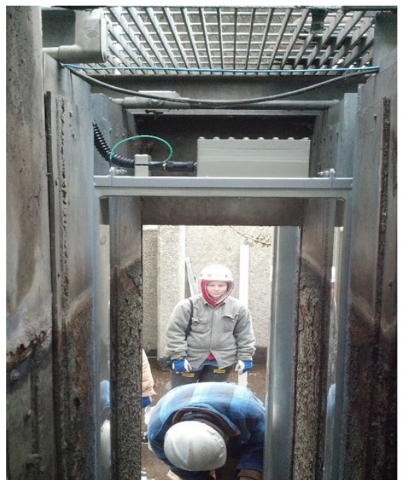
South Ladder Upstream antenna. ID. 01
