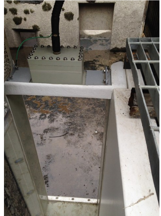
Upstream ladder antenna. ID. 01
