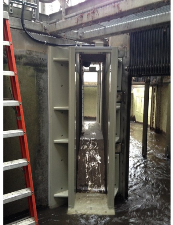
North Ladder Upstream antenna. ID. 03
