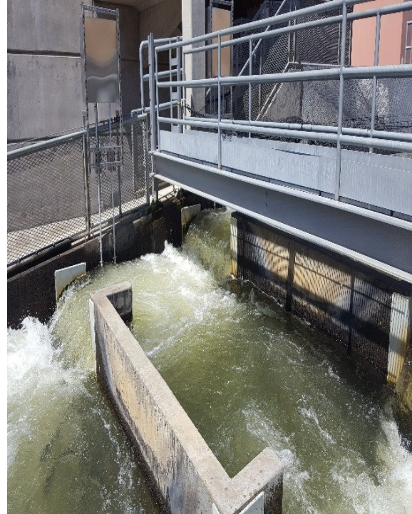
Figure 8. JO2 antennas after water up.
