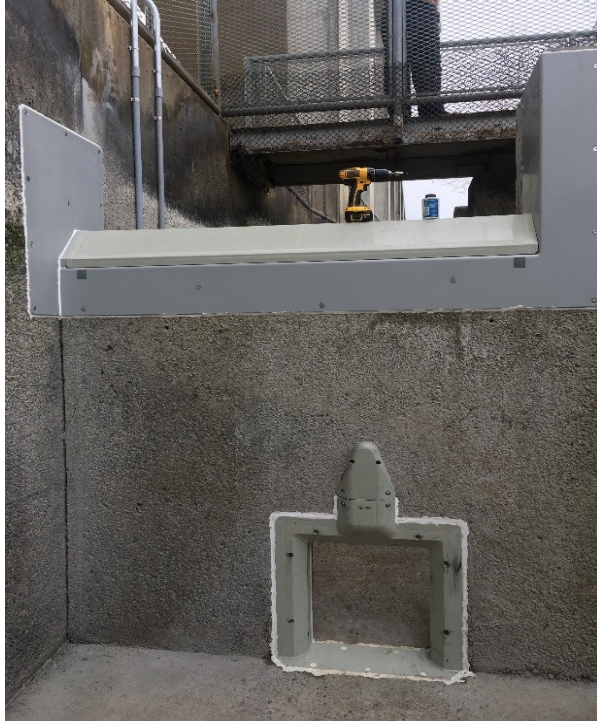
Figure 7. JO1 antennas before water up.
