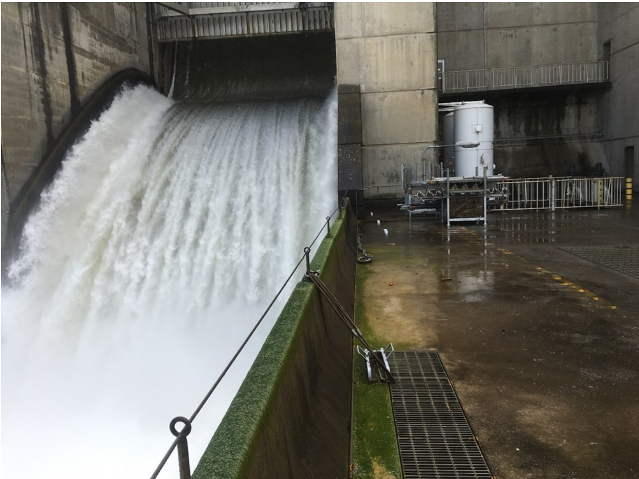
Figure 6. Lower Granite Spill Bay # 1. Proposed location for the OGEE antenna installation. CONTINUED →
