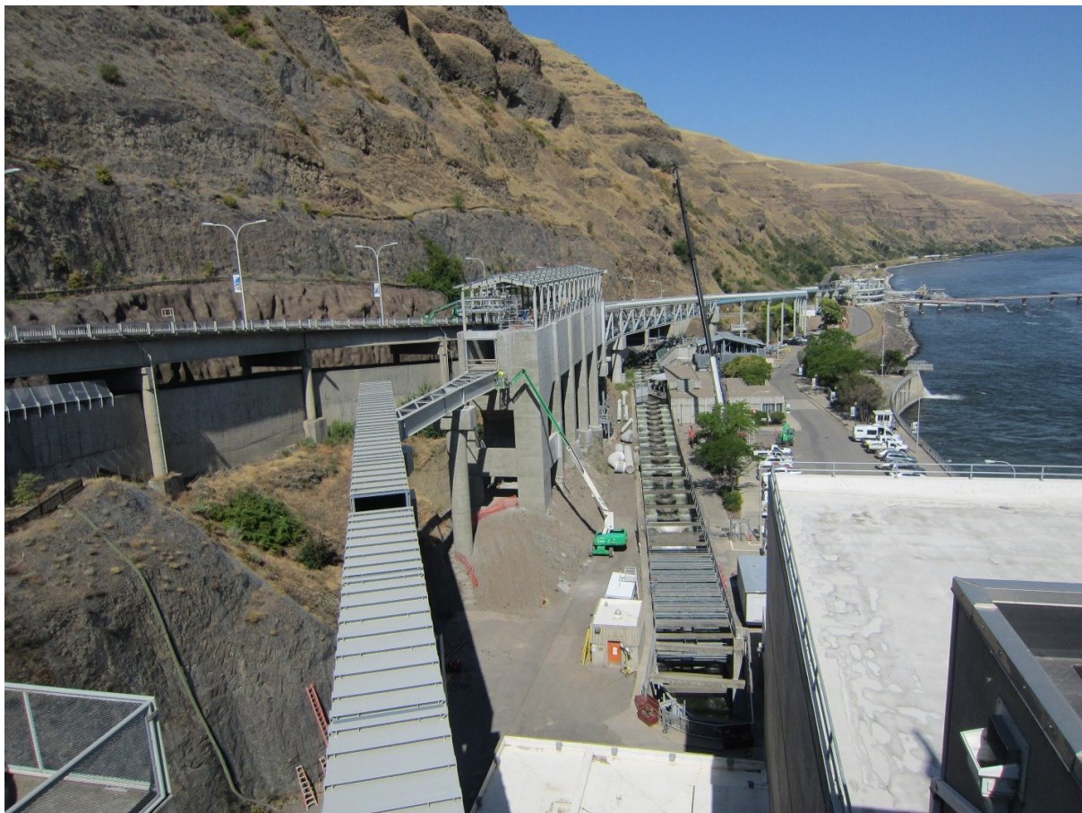
Figure 9. Lower Granite Juvenile Bypass reconstruction.
