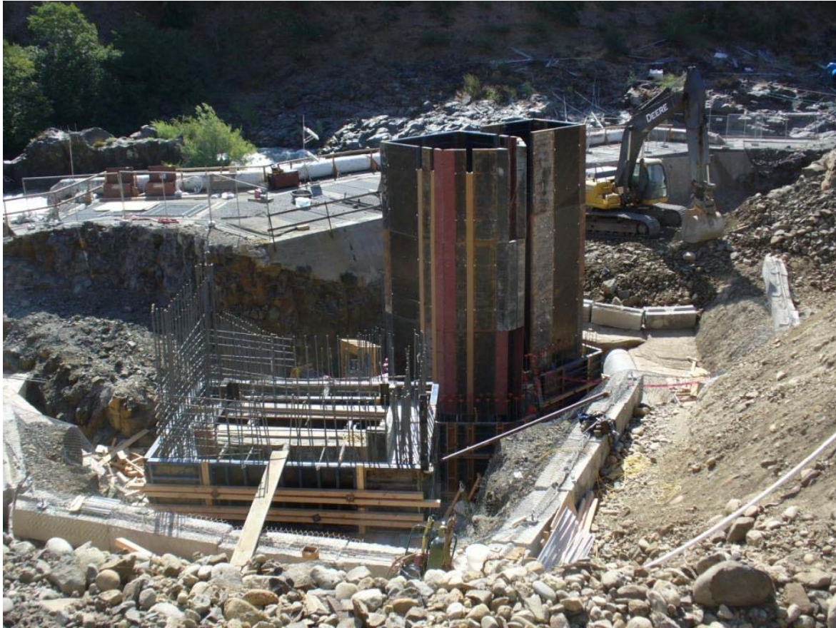
Figure 4: Construction on the Klickitat River Project
