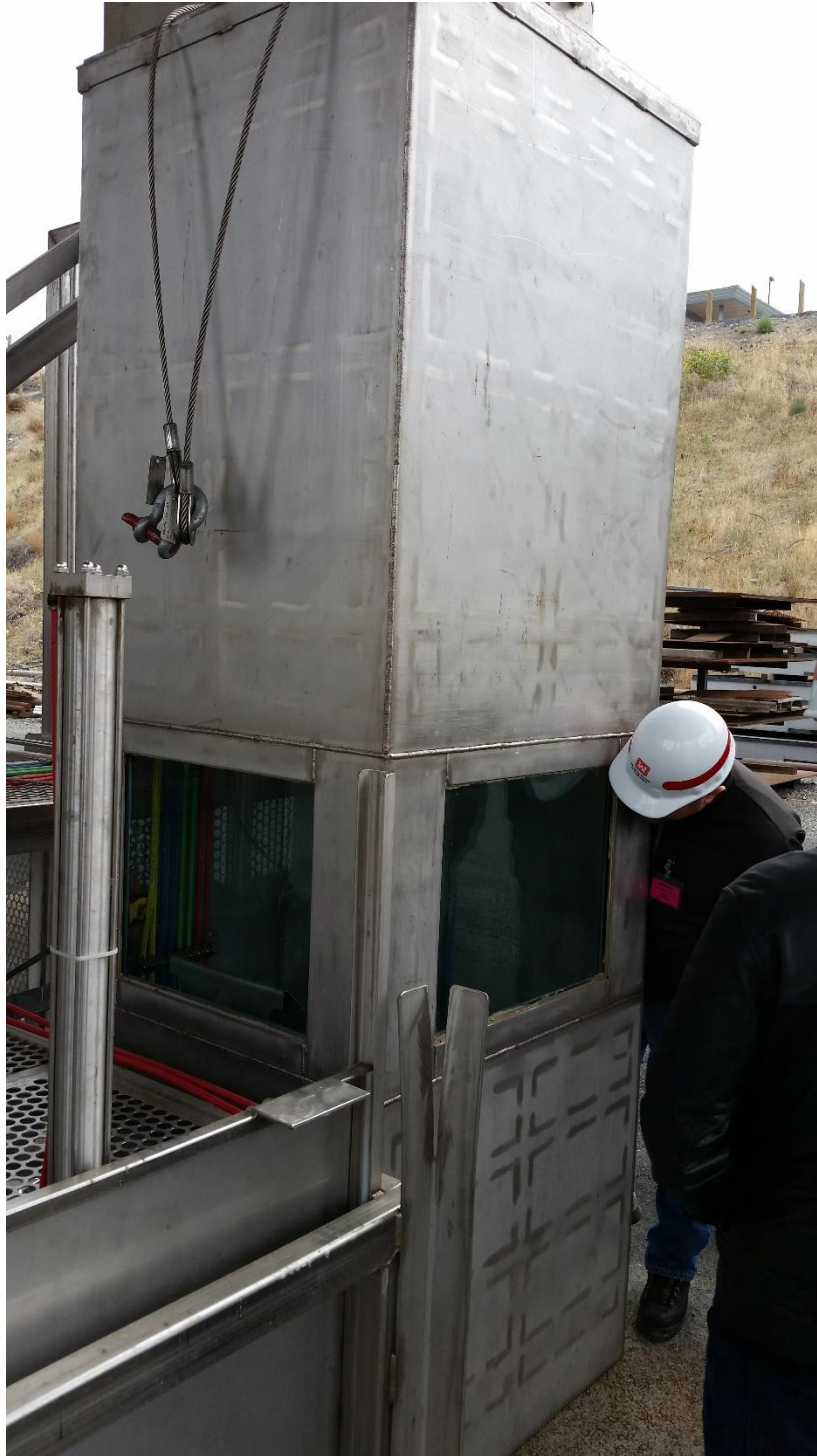
Figure 8. Manual SbyC System at Ice Harbor South Shore Ladder
