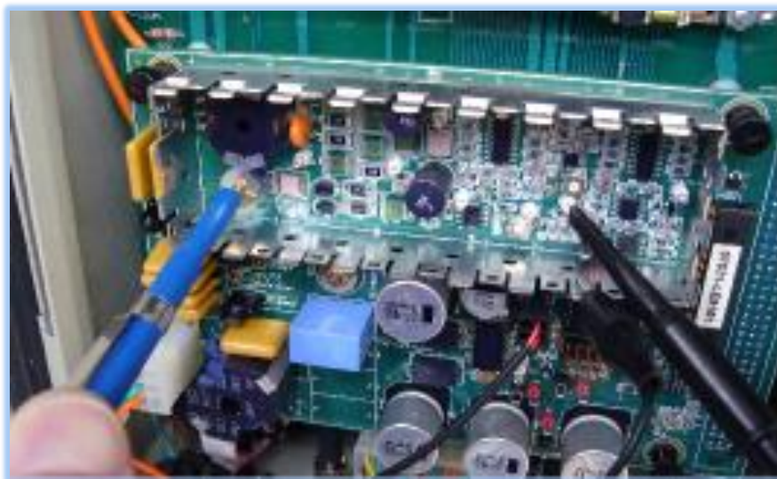
Figure 9. PTAGIS staff repairing a transceiver device.
