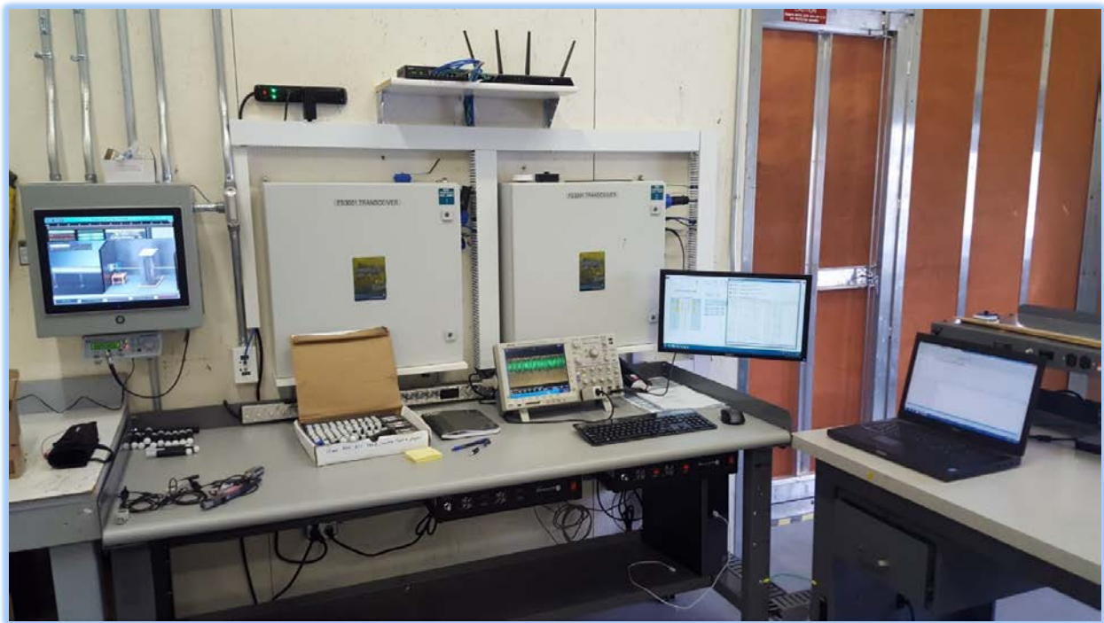
Figure 27. BCC Simulator transceivers, external HMI, and other equipment
