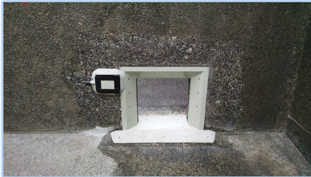
Figure 10. New orifice antenna installed in Lower Granite Adult Ladder
