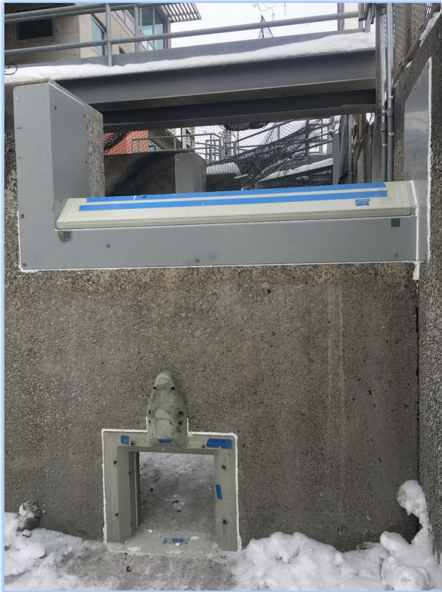
Figure 11. New overflow and orifice antennas installed at North Shore John Day Ladder
