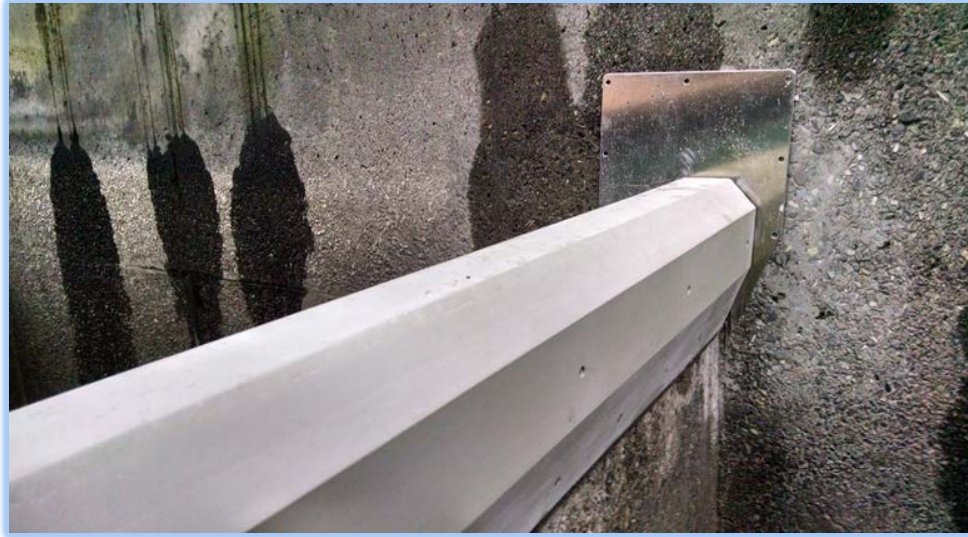
Figure 9. New overflow antenna installed in Lower Granite Adult Ladder
