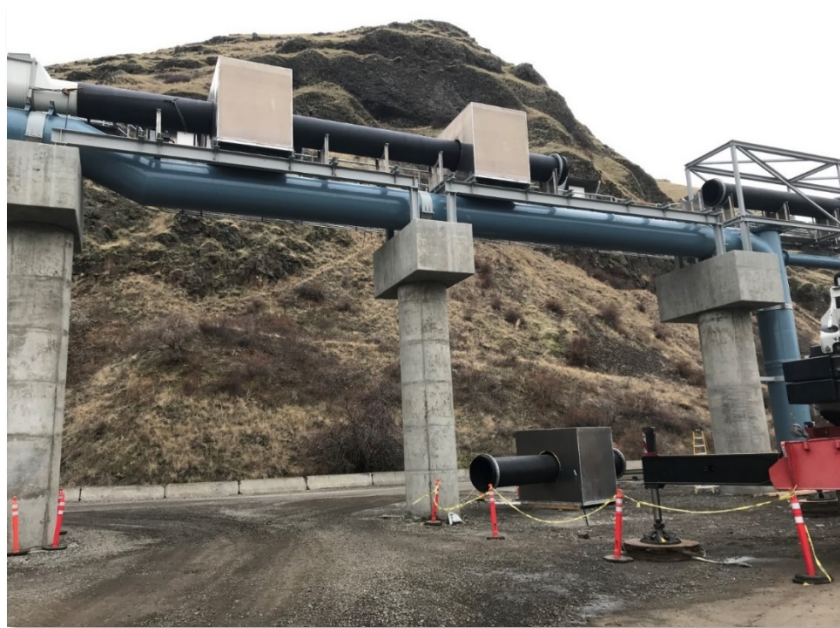
Figure 13. Lower Granite Juvenile Bypass Construction
