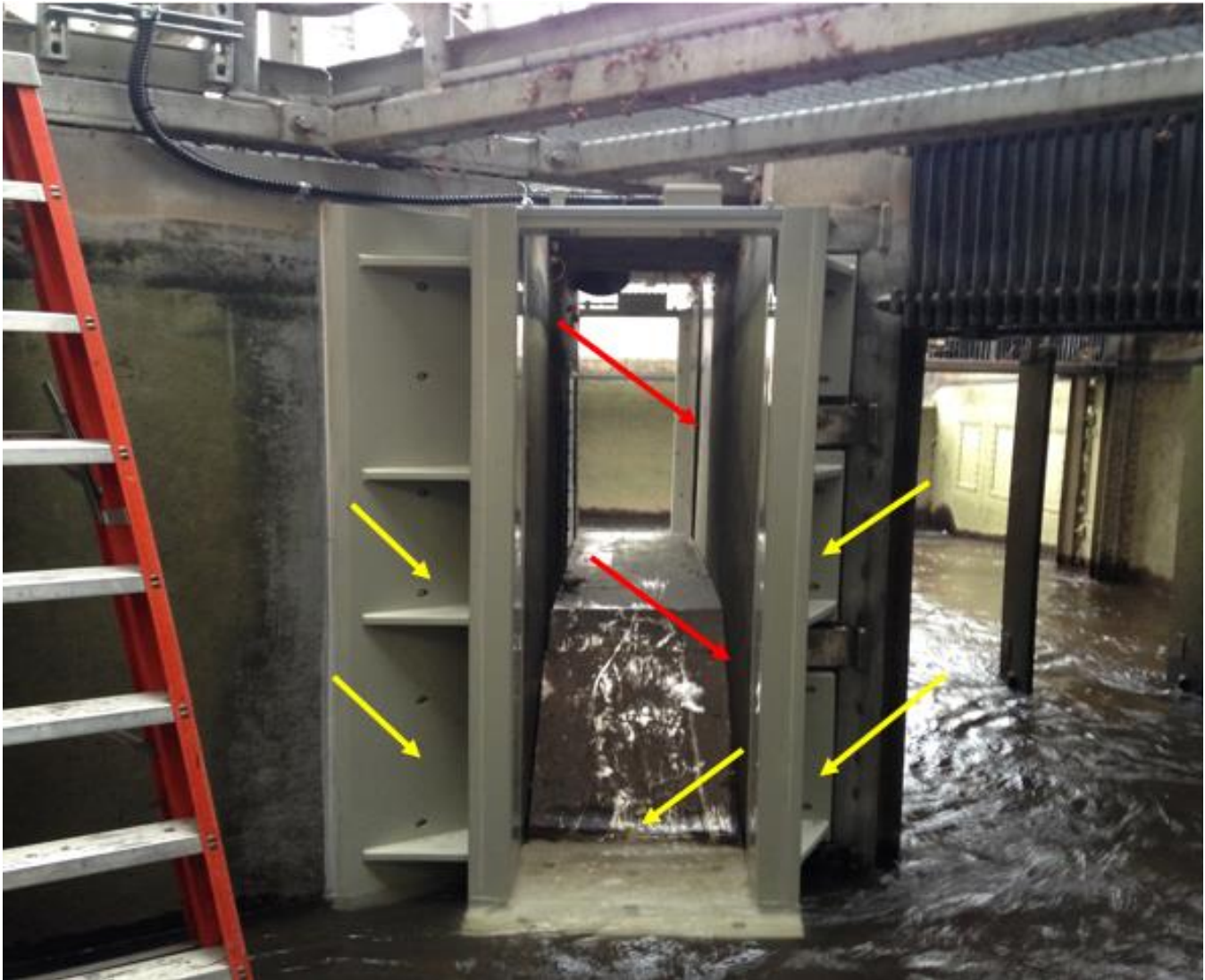
Picture 3. LMA north Counting Window antenna
