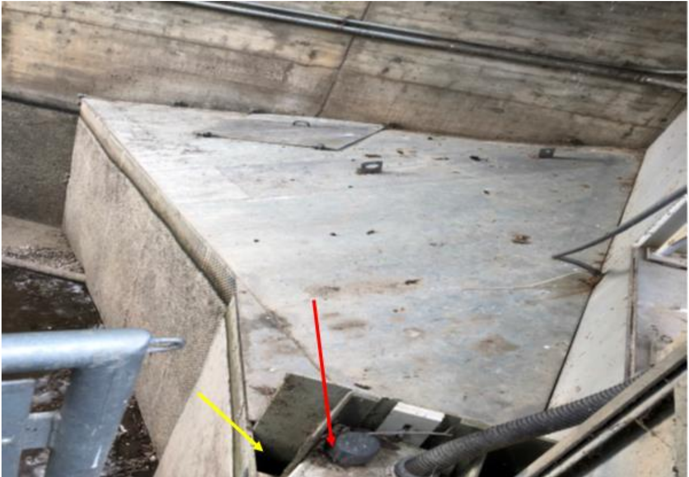
Picture 5a. MC1 Spacer section where lamprey have become entrained.
