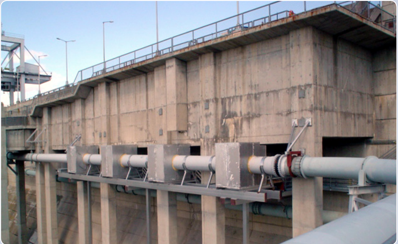
The new PIT tag detectors located on the Full Flow Bypass pipe at Ice Harbor Dam.
