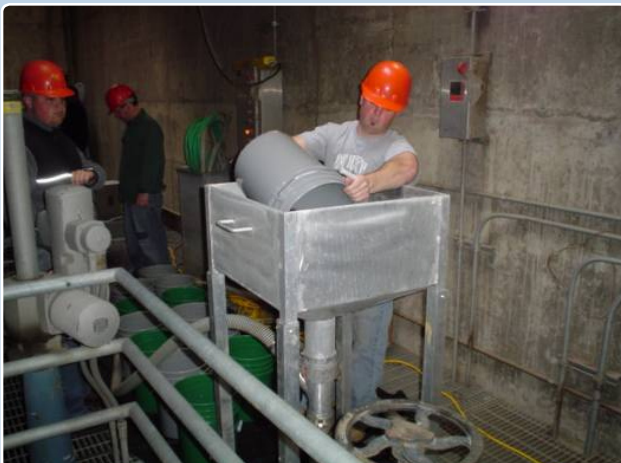
The hopper and flexible hose used for releasing fish at Ice Harbor Dam.
