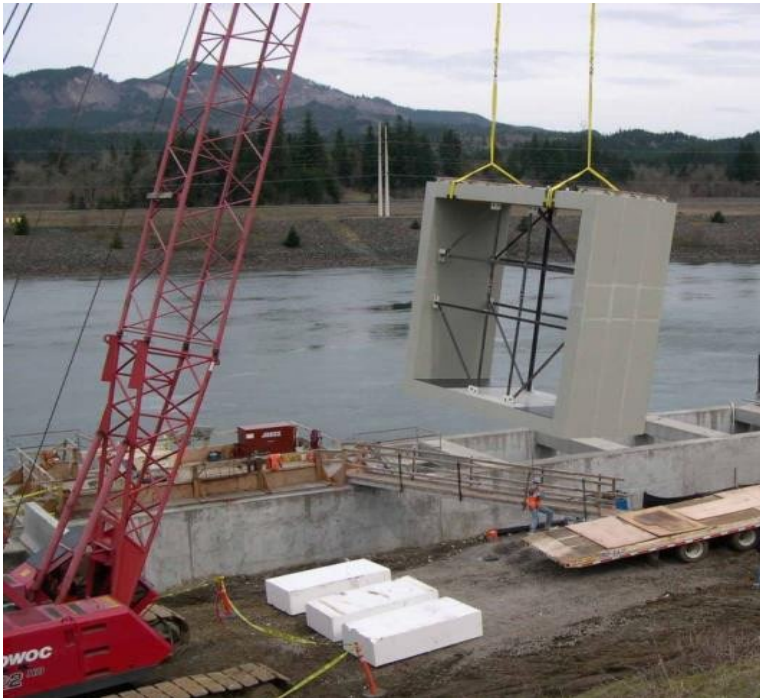
Figure 1. PIT tag antenna being lowered into place at the corner collector flume at Bonneville Dam, 2006.
