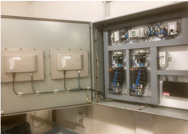
Figure 5. Complete DCP in one enclosure.
