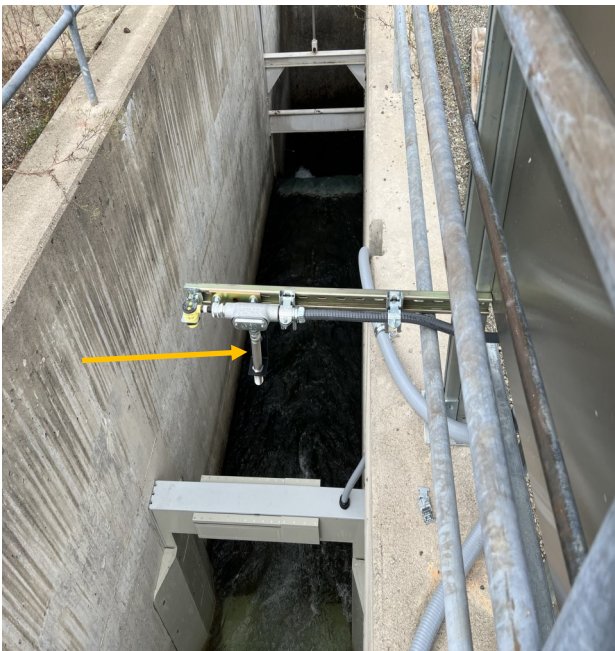
Figure 7. Level and Temperature Sensors.
