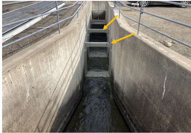
Figure 6. Antennas in fishway.
