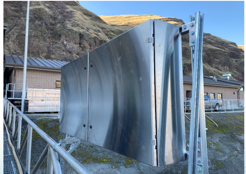
BLL panels installed at GRJ
