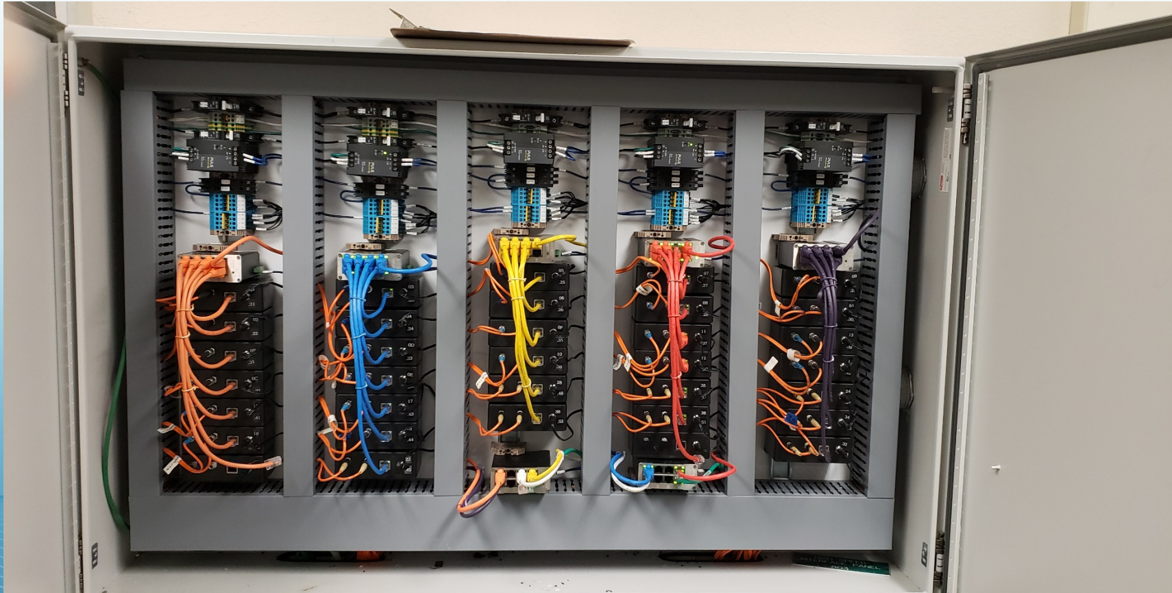
BO3 Completed STE Panel
