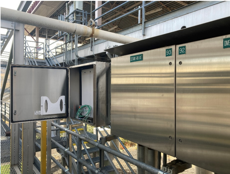
BLL panels installed at LMJ
