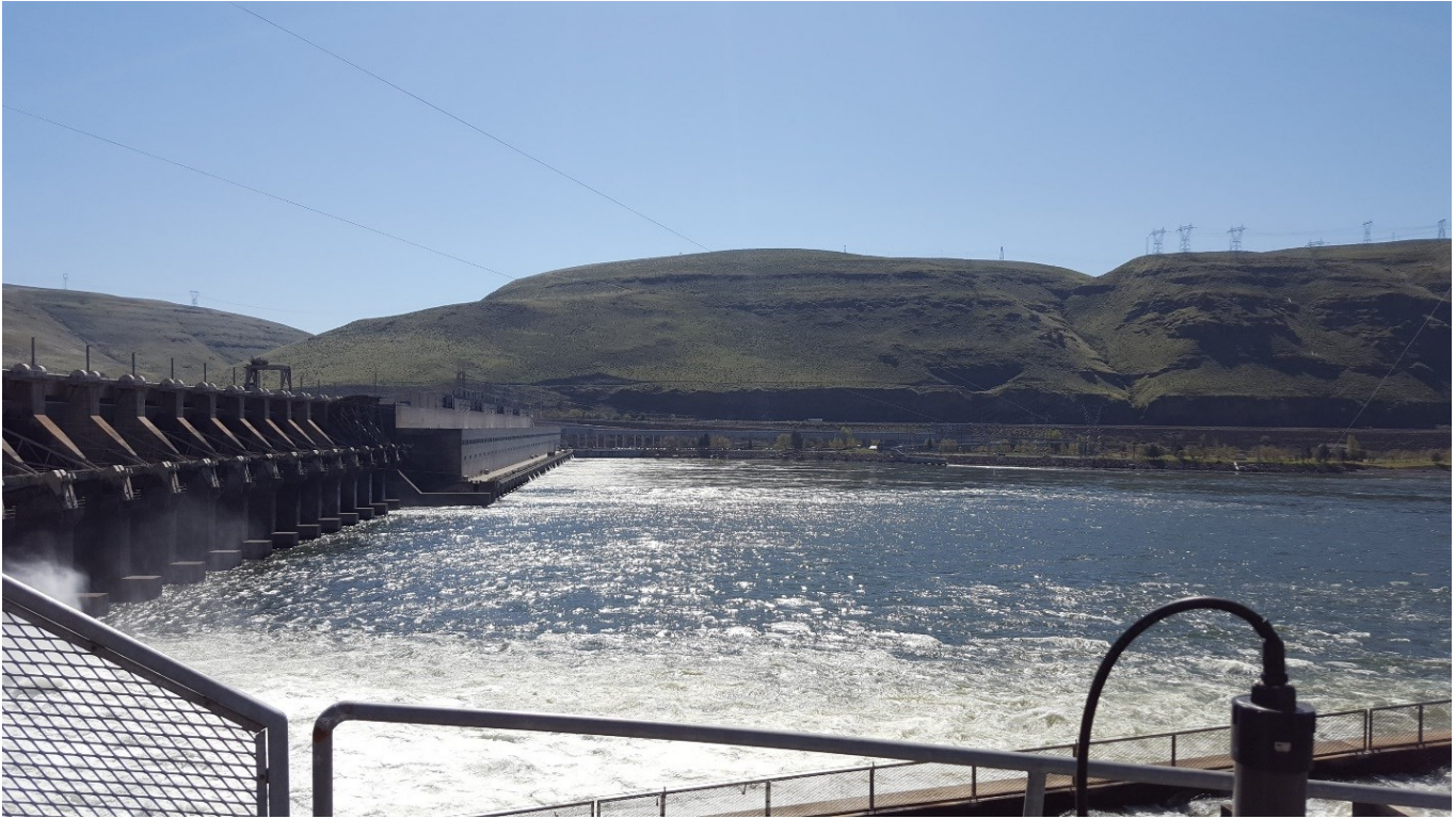
John Day South Ladder Viewed from the North
