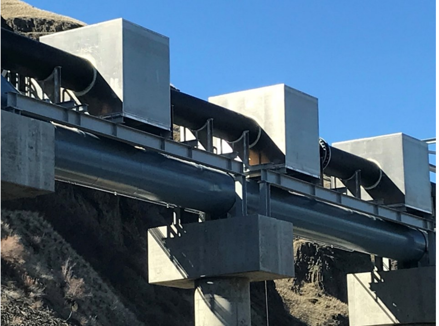
Figure 6. New Full Flow System at Lower Granite Dam
