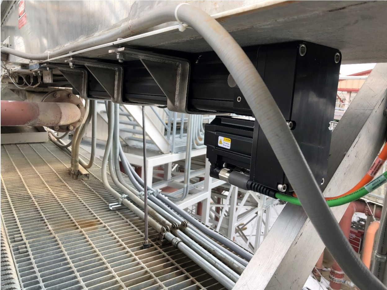
Figure 5. New Electric Cylinder at LMJ B-Side Gate.
