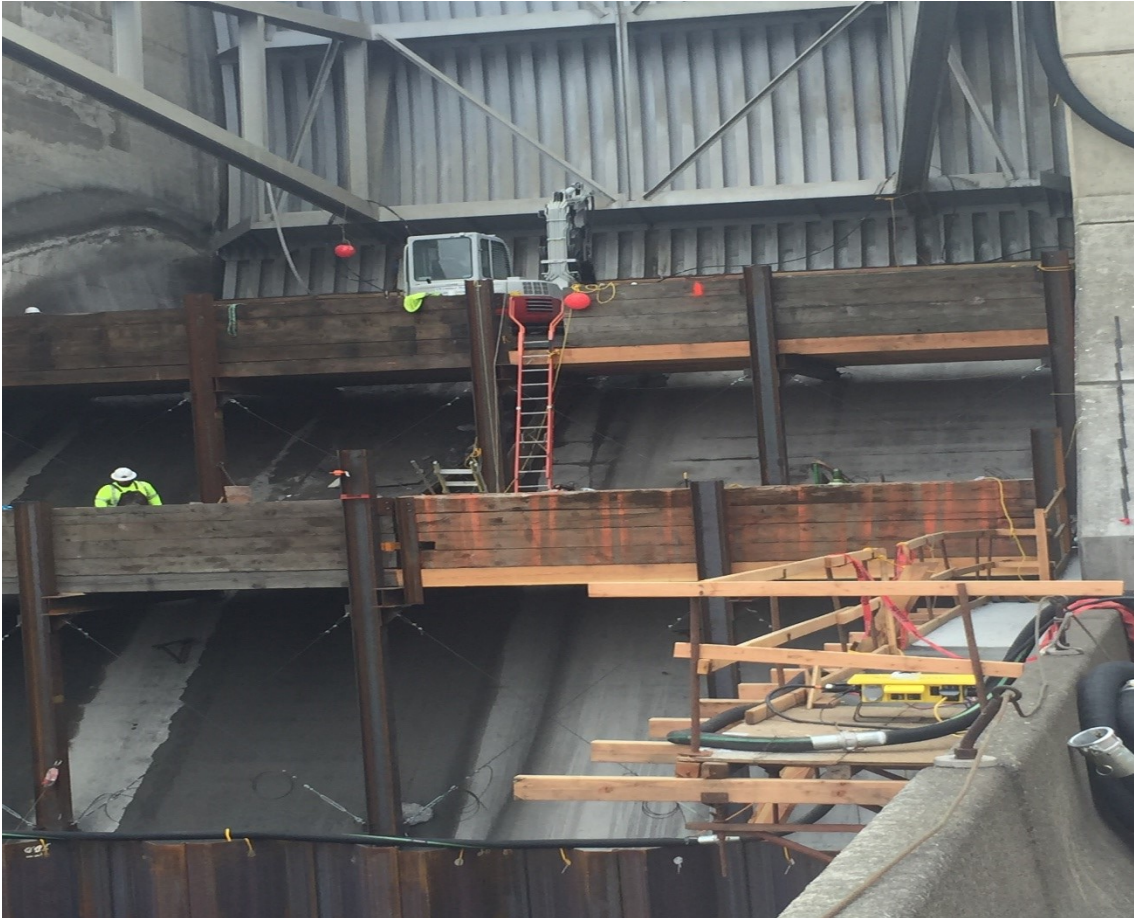
Figure 1. October 2019. GRS Spill bay # 1 under construction. Phase 1: Concrete removal.
