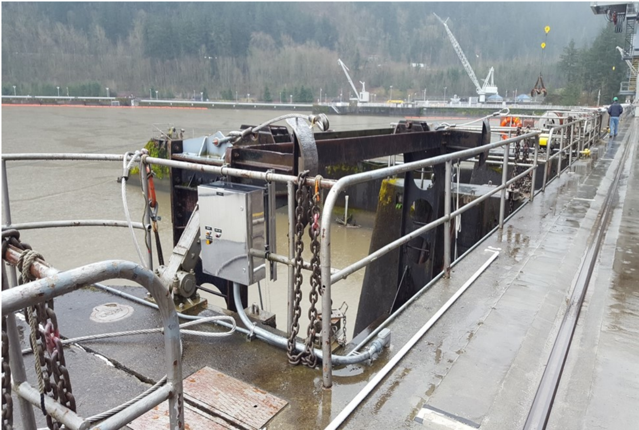
Figure 4. Bonneville Dam Powerhouse 1 Intake Deck.
