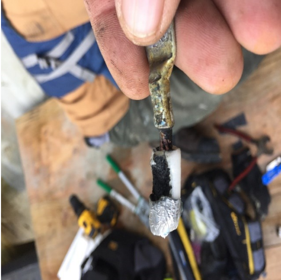
Figure 6. Antenna cable end damaged by electrical arching.
