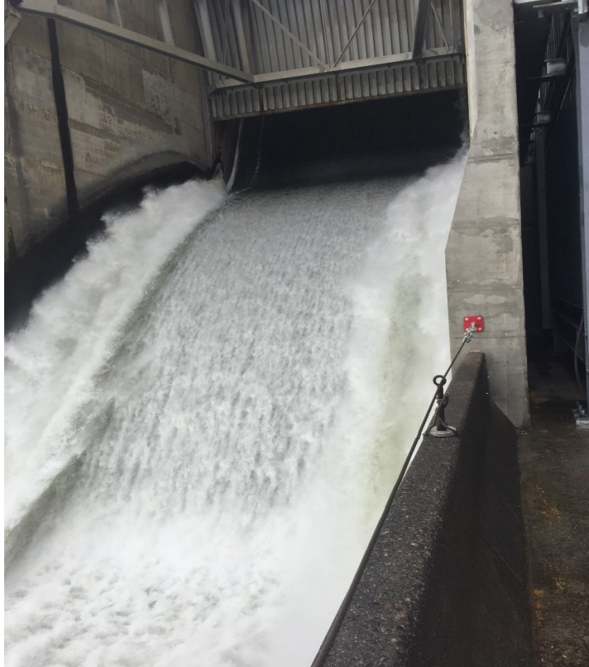
Figure 5. Lower Granite Dam Spill bay # 1, PIT tag detectors in operation and detecting tags, May 2020.
