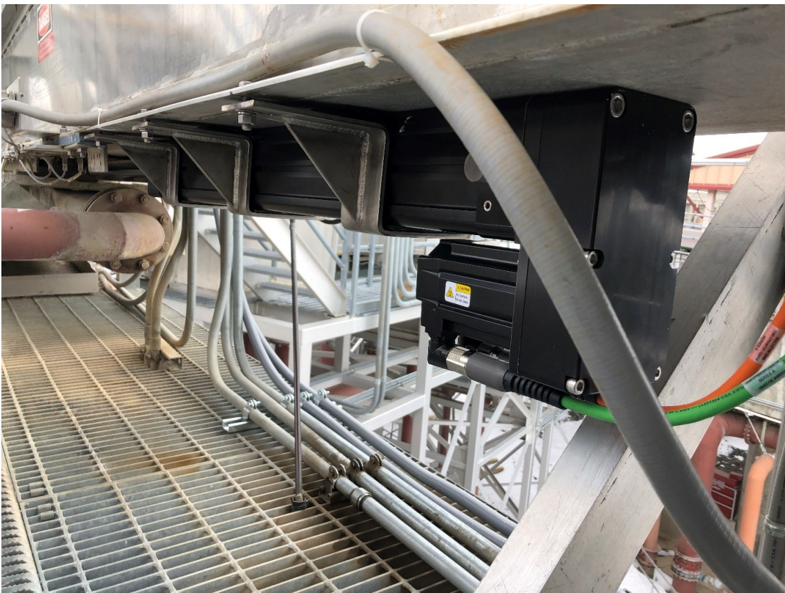
Figure 4. New electric cylinder at Lower Monumental Dam Juvenile Bypass Facility B-side gate.
