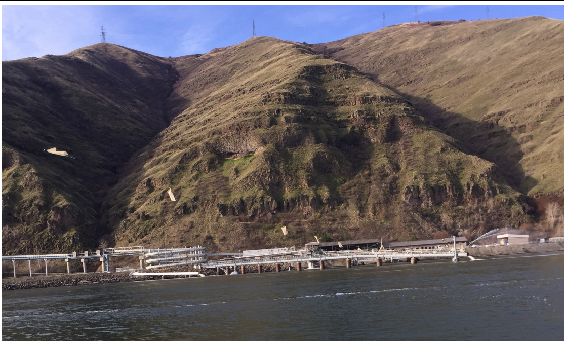
Figure 2. Lower Granite Juvenile Bypass Facility
