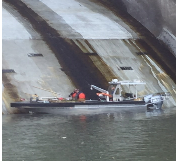
Figure 7. Work skiff providing access to the OGEE.
