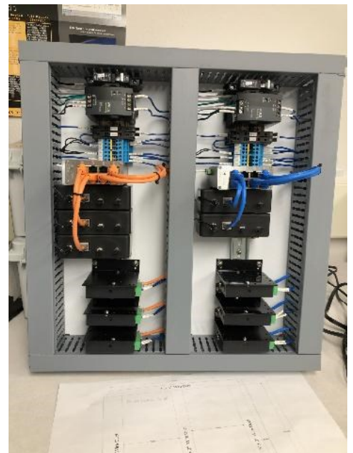
Figure 3. Upgraded communications panel ready for installation at PRO.
