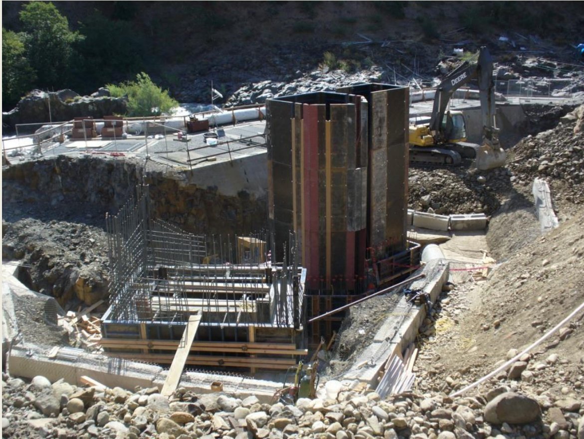
Figure 19 - Construction on the Klickitat River Project
