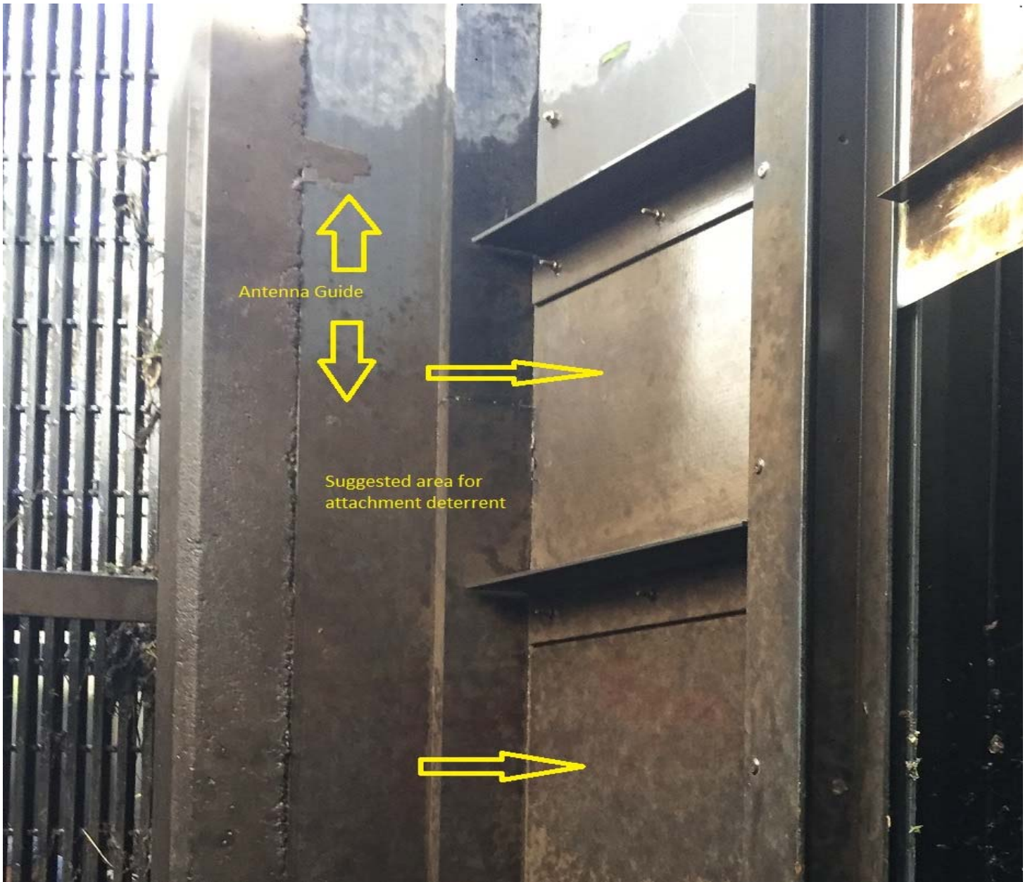
Picture 2 and 4. Downstream area of counting window, upstream side of antenna guide.
